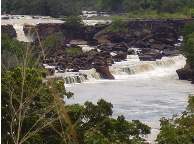
Malagarasi Hydropower Project Site
