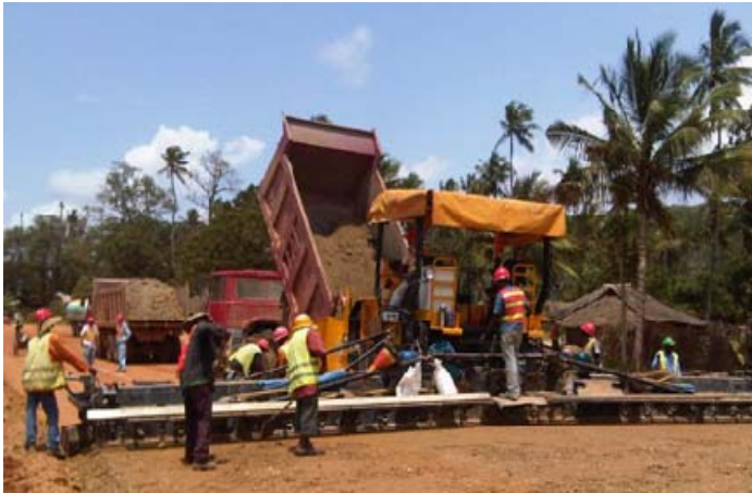
Laying of C-1 layer on Tanga-Horohoro road at KM 41 + 200 17 Sept 2011
